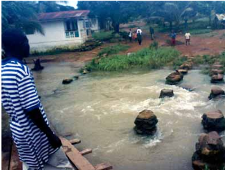
This bridge was built by the local people but washed away in the recent rains
